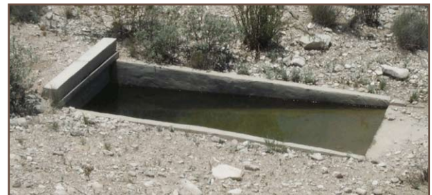
Figure 8. Underground storage tank (above) and trough (below) for concrete catchment.
