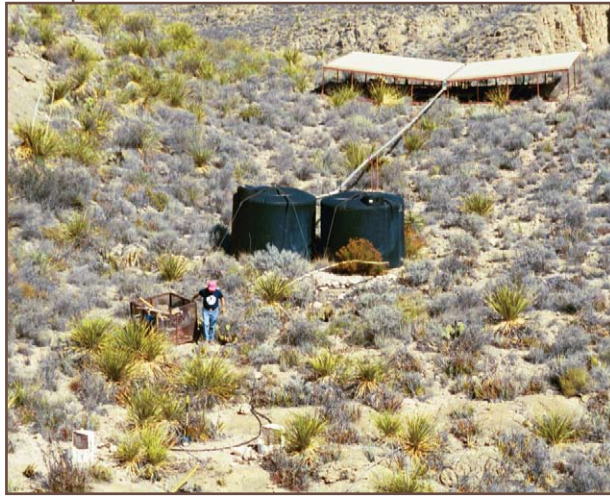
Figure 3. A Black Gap Guzzler rainwater catchment.
