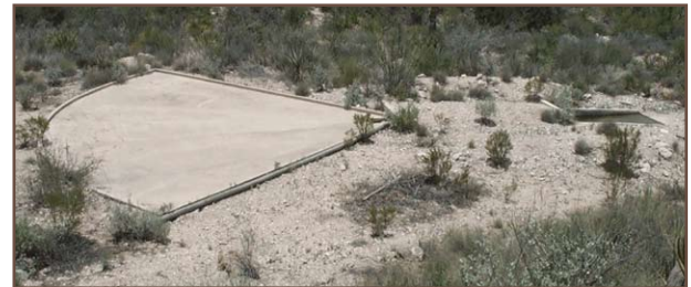
Figure 8. Underground storage tank (above) and trough (below) for concrete catchment.
